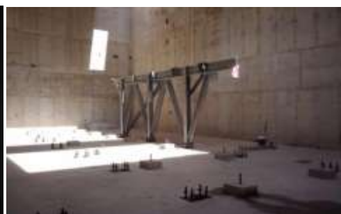
Assembly of car dumpers
